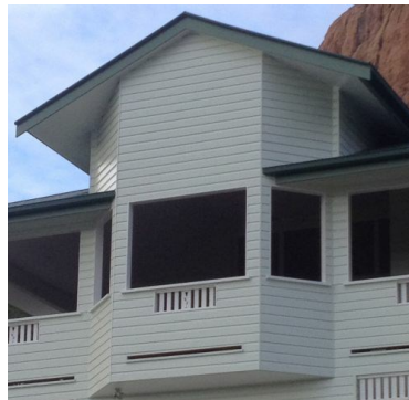
Figure SC6.2.3.21 Illustrates new works using manufactured cladding in imitation of traditional lightweight materials
